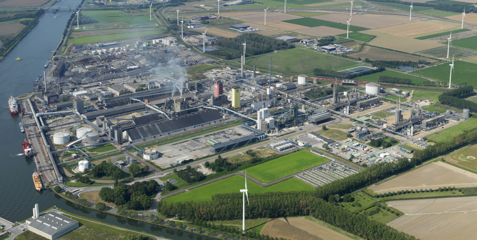
Overview of Yara Sluiskil
